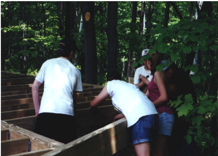
Students working with local architect and contractor to build amphitheater stage.
